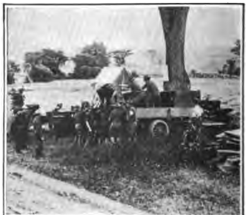
④ Underwood & Underwood, New York UNLOADING BAKE-OVEN EQUIPMENT AT CAMP WHITMAN, BEEKMAN, N. Y.
